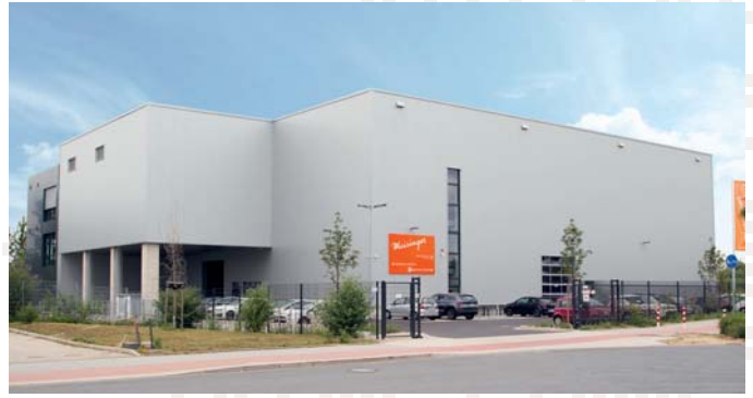
MEISINGER Headquarters Neuss, Germany
