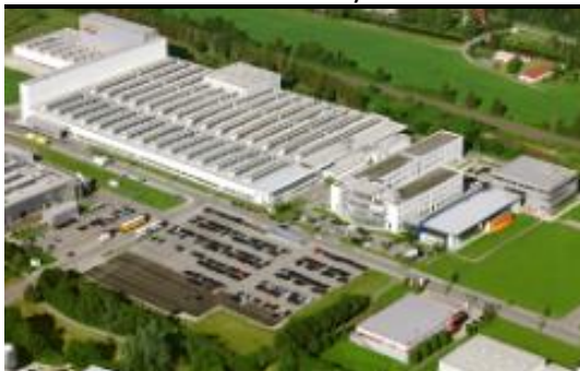
Handtmann Maschinenfabrik with technology center
