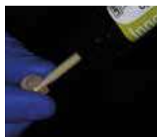
17. Cement application in the intrados
